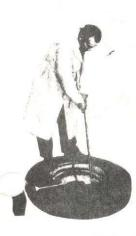
1. Remove valve core to deflate and loosen tire from bead seat of rim on both sides. Lubricate upper bead of tire thoroughly. With stops toward rim, insert spoon ends of both tools about 10 inches apart. While standing on tire to hold bead in well, pull one tool back toward center of rim. 2. Hold first tool in position with one foot and pull second tool toward center of rim. Progressively work top bead off rim, taking additional bites if necessary.
