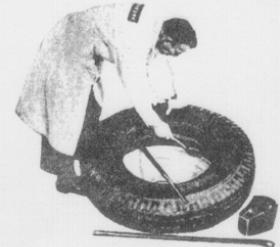
3. Lubricate last section of lower bead to facilitate mounting.
