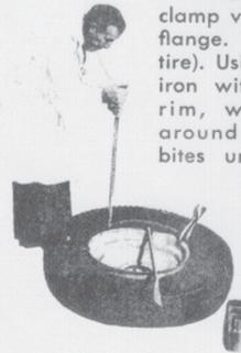
6. To get top bead in place stand on tire and force bead down as far as possible and clamp vice grip pliers on the flange. (snub side toward tire). Using spoon end of tire iron with lug side towards rim, work progressively around bead using small bites until bead slips over flange onto rim base. In order to mount last 6" of bead it usually is necessary to insert second tire iron and lubricate the last bead portion.
