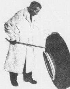
3. Stand tire and tube in vertical position with valve at top of assembly and remove valve from valve hole. Then place valve at bottom of assembly and pull out upper portion of tube so it will not interfere with demounting the second bead. Lubricate second bead. At top of assembly insert straight end of tool between bead and back flange of rim at about a 45° angle. Turn tool so it is perpendicular to rim. Pry second bead off.
