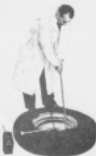
1. Remove valve core to deflate and loosen tire from bead seat of rim on both sides. Lubricate upper bead of tire thoroughly. With stops toward rim, insert spoon ends of both tools about 10 inches apart. While standing on tire to hold bead in well, pull one tool back toward center of rim.
